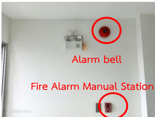
Alarm bell & Fire Alarm Manual Station
